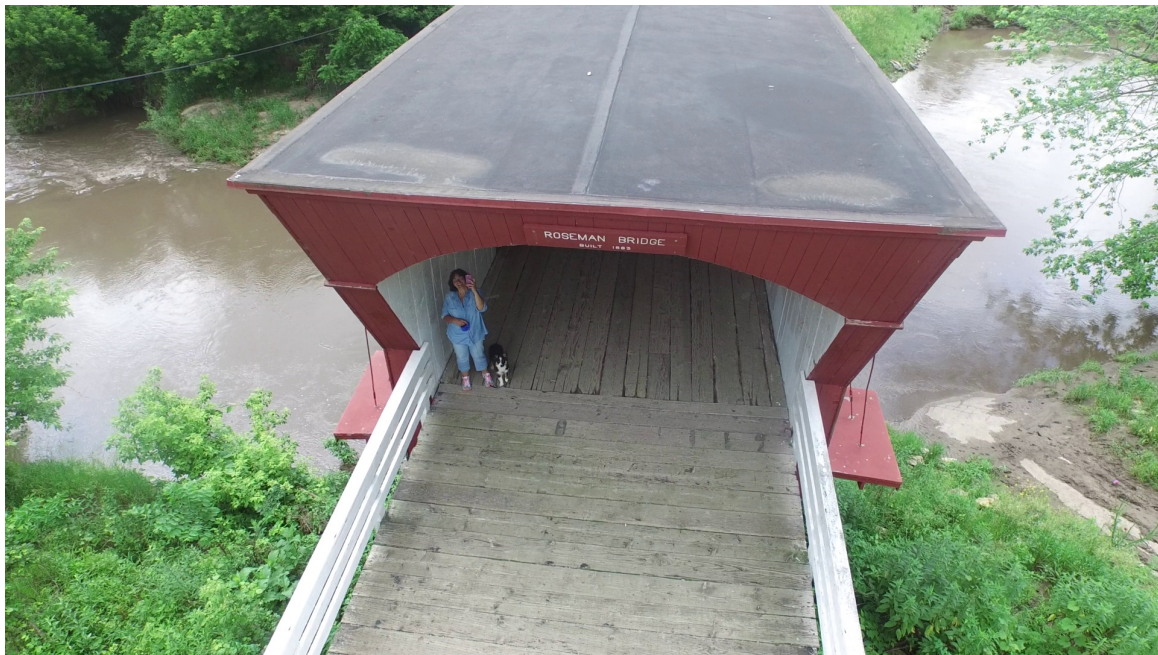
FIGURE 65: Roseman Bridge sequence, frame 25
