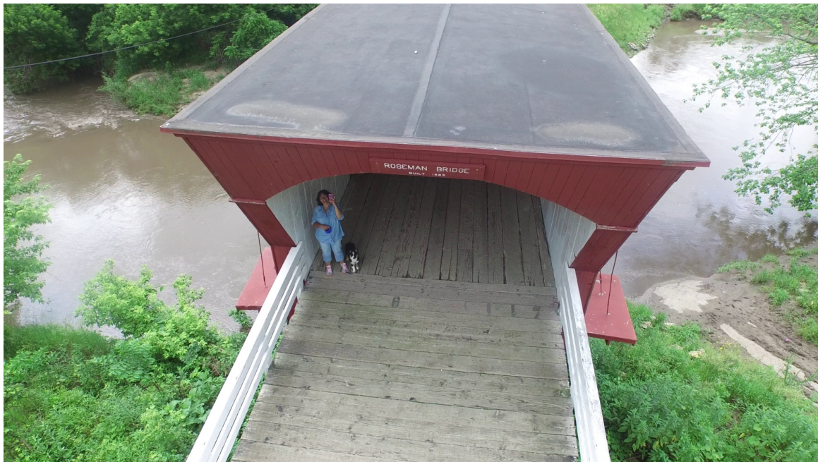
FIGURE 41: Roseman Bridge sequence, frame 25
